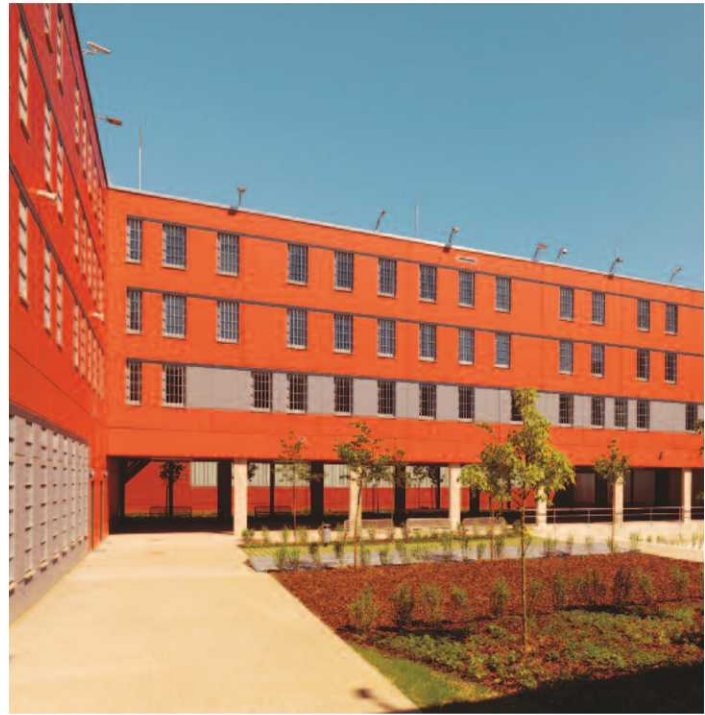
Lighting of exteriors and walkways can be easily controlled with GAMMA instabus .
