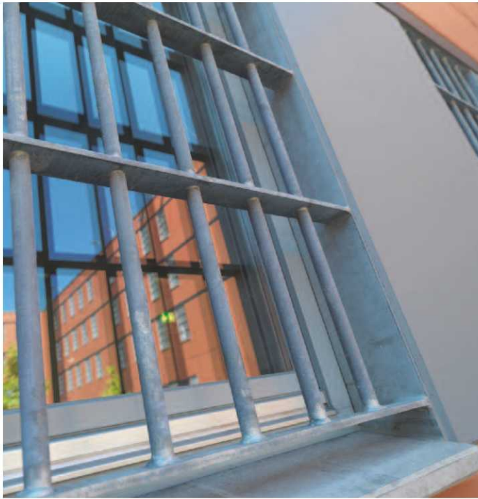
Windows left open accidentally can be identified and closed before they pose a risk.
